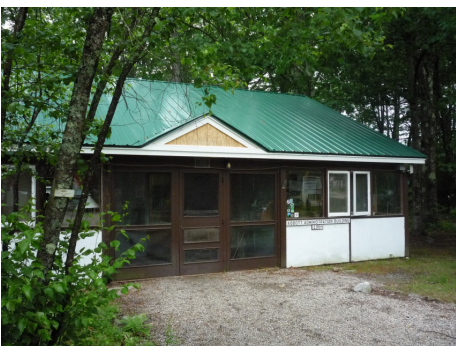
New Roof for the Abbot Administration Building
