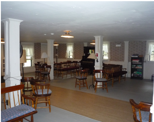
Repairs and Fresh Paint for the Lobby at the Inn
